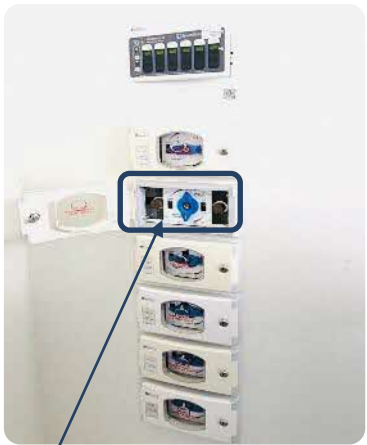
N 2 O pipeline supply switched off in NUH Medical Centre OT
